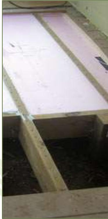
*Friction-fitted rigid slab insulation*
