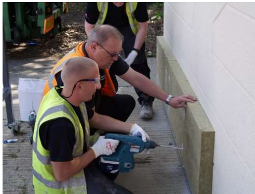
Fitting cladding (left) and external render (above)
