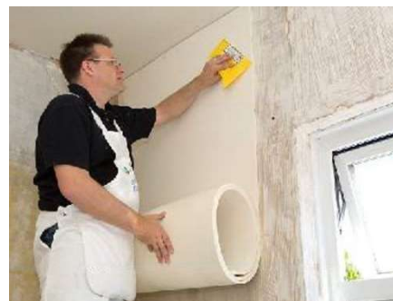
Fitting Sempatap Thermal (shown on a wall but can be used on ceilings)
