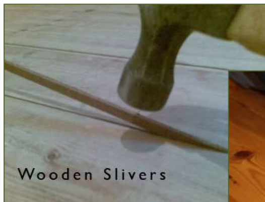
Filling cracks in floorboards with wood and rubber strips
