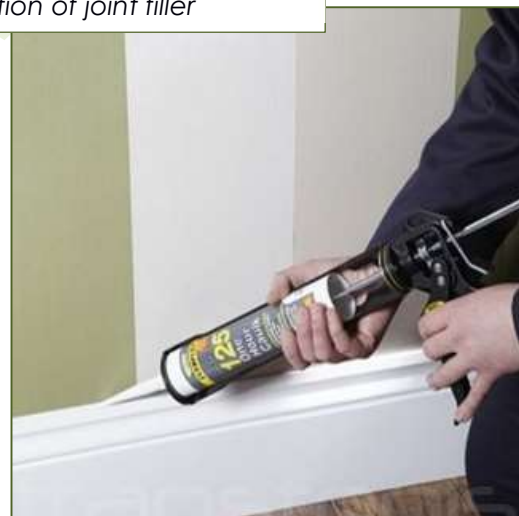
Examples of a door curtain and application of joint filler
