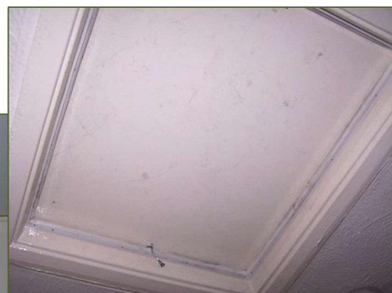
Cracks between wall and ceiling and draught-stripped loft-hatch
