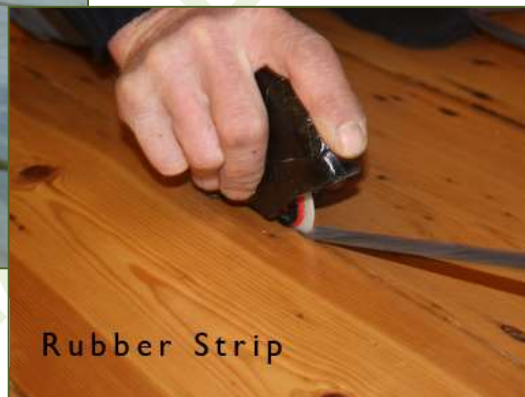
Filling cracks in floorboards with wood and rubber strips
