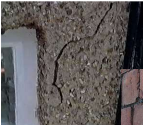
Cracked render and damaged pointing
