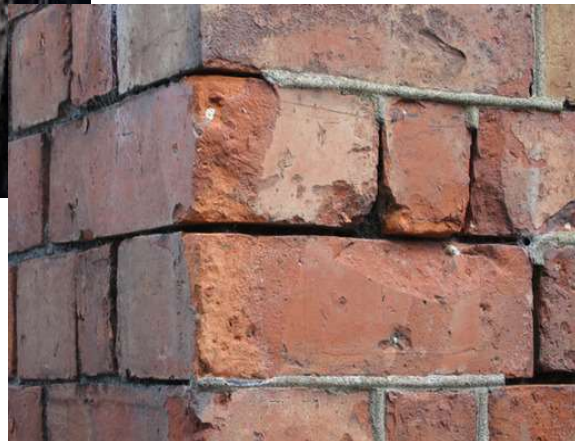
Cracked render and damaged pointing
