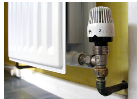
Figure 3 Thermostatic radiator valve
