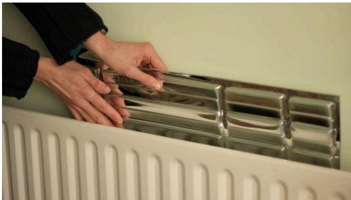
Figures 4 & 5 Fitting an insulated radiator panel
