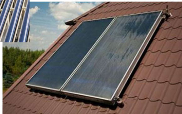
Roof-mounted solar thermal energy panels: evacuated tube collectors (above) and flat plate collectors (right)
