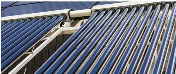
Roof-mounted solar thermal energy panels: evacuated tube collectors (above) and flat plate collectors (right)
