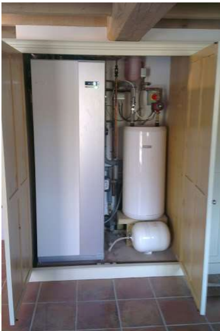
Typical GSHP internal installation (left) and ASHP external unit (right)
