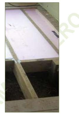
Friction-fitted rigid slab insulation
