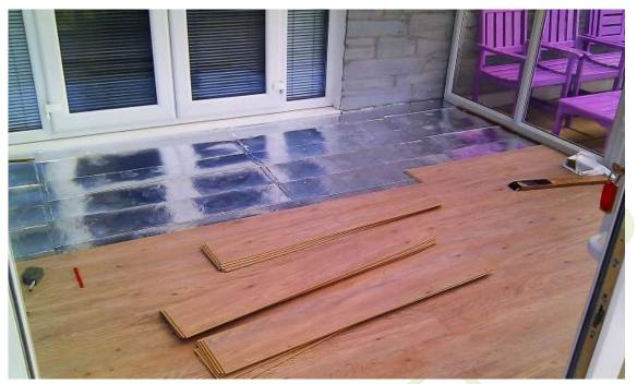
Example of insulation under laminate floor and a thin flexible insulation product on a roll (image shows 6mm Palziv product) Image courtesy of http://www.palziv.com/Thermal insulation.html
