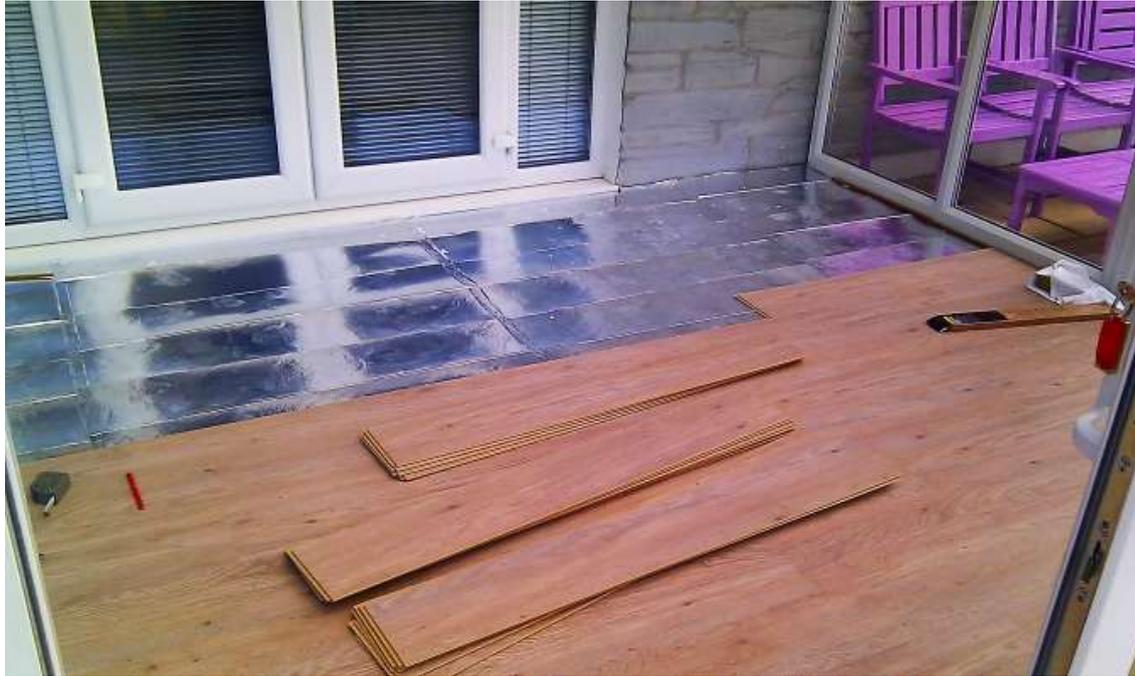
Example of insulation under laminate floor and a thin flexible insulation product on a roll (image shows 6mm Palziv product)
