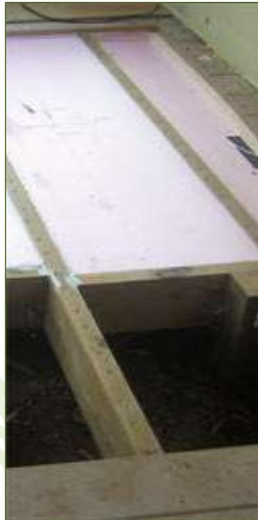
*Friction-fitted rigid slab insulation*
